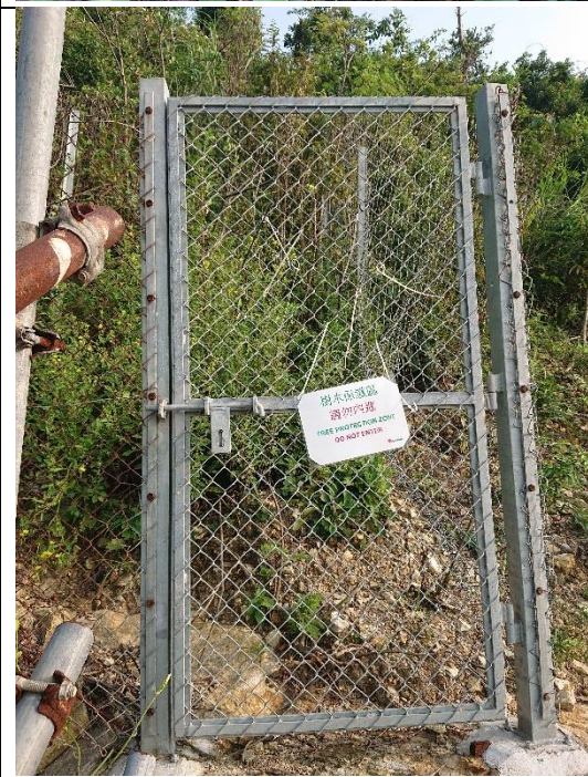
Photo 2 – Current situation of fencing and warning sign
